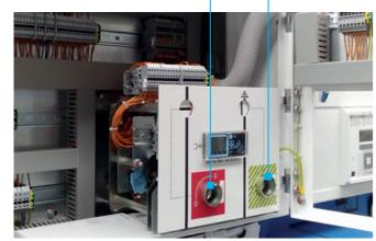
Mechanically interlocked earth switch and LBS with panel cover
