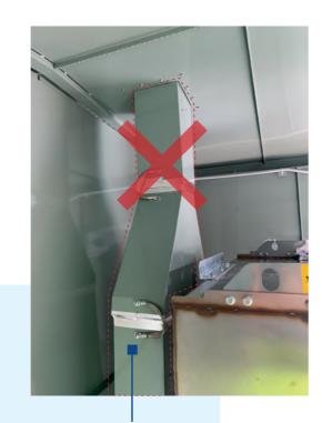
The need for gas chimneys is eliminated with DF2+, saving cost, space and simplifying installation
