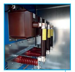
Fuses can also be used for protection instead of the VCB
