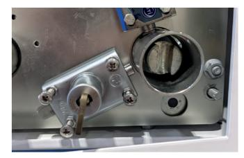
Ronis key interlock fitted to LBS/ESW panel
