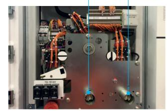
Mechanically interlocked earth switch and LBS without panel cover
