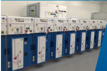
The example to the left shows a DF-D-EDN panel with a hinged door front mounted protection relay compartment. Above it is a horizontally mounted DF-LKB
