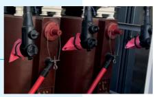
Plug-in bushings with earth screened HV terminations
