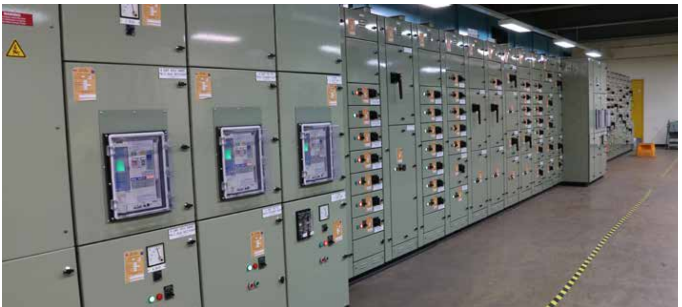
Above: Terasaki AR ACB retrofit from Stanwell powerstation QLD
