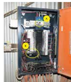
Above: Arc flash damage to the low voltage switchboard showing the isolator in the "On" position (A) and the circuit breaker that was to be removed (B).
